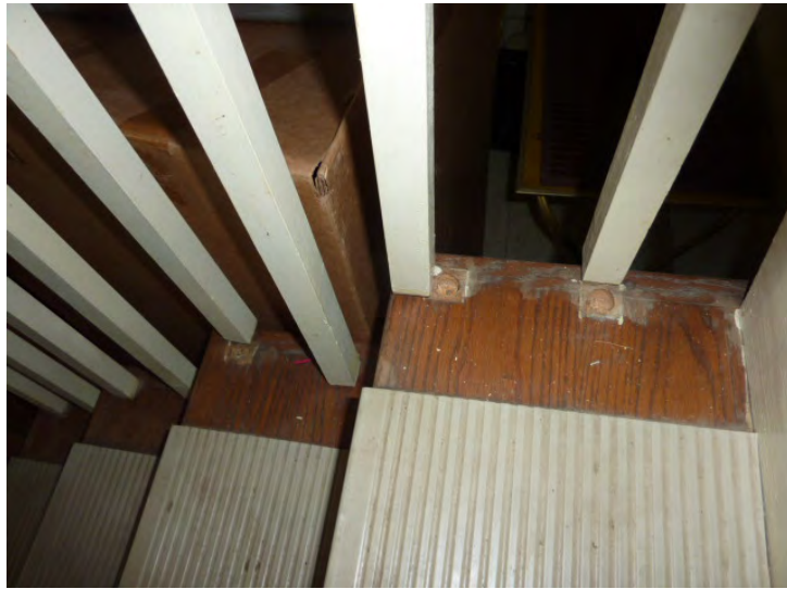
Stair balusters have sheared off and should be replaced. Worn vinyl treads should be replaced.
