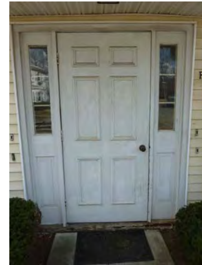
Entry doors and storm doors are well worn and shown to be replaced. Concrete cracking due to rusting reinforcing at door threshold is shown to be repaired in Year 1.
