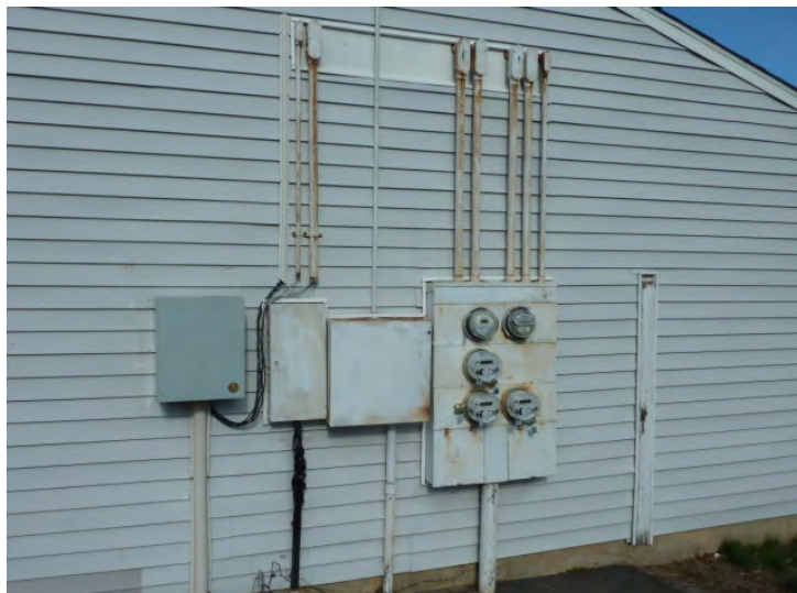
Electric meters, alarm and cable box is shown to have a weather-tight enclosure constructed at each building in Year 1.
