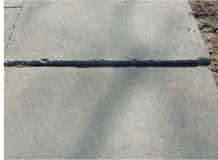
Typical trip hazard at concrete walks and stoops should be eliminated.
