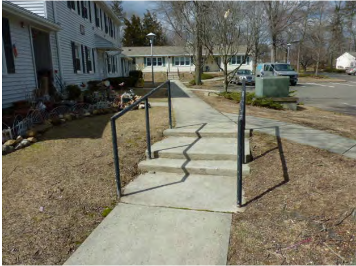
Concrete walks site-wide are in generally fair condition. Proper steel pipe handrails should be installed at site stairs site-wide.
