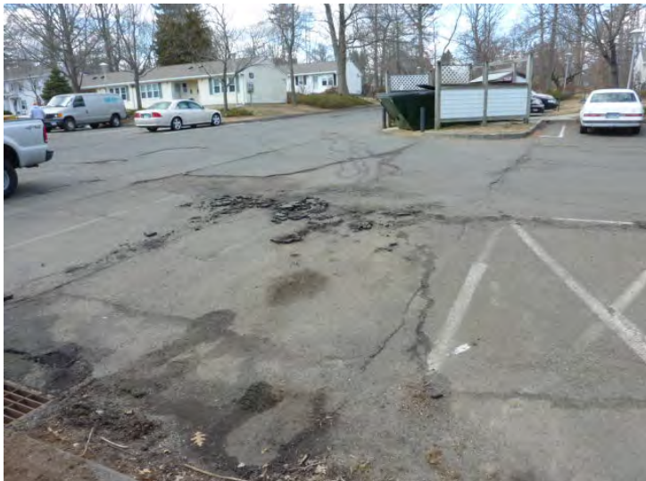
Severe cracking in asphalt paving at sub-base failure.
